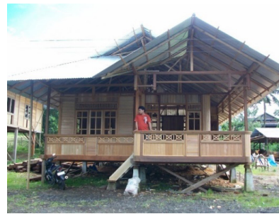
Figure 8. Minahasa vernacular house in Woloan village, Tomohon. The roof variations with the addition of a shield form to cover the part of the terrace, and the number of stairs on the front which only has one ladder (Photo by Ronald 2019)
