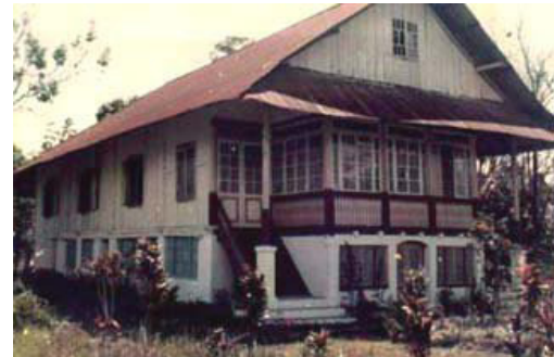
Figure 4. Houses with poles and under space made from concrete (Photo of Bode Talumewo Repro by Ronald Kolibu 2019)
