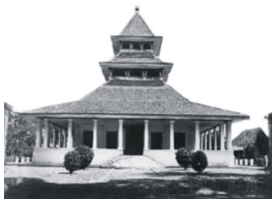
Figure 7. A traditional mosque in Bandung West Java with a three-level 'meru' or mountain-like roof. The peak is pyramid-shaped composed of four triangles called nyungcung (kitlv.nl, 1920)
