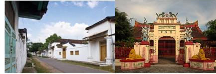
Figure 3. Chinese houses and Cu An Kiong temple in Lasem (source: survey, 2015)
